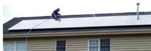
Solar Service installer performs last hook ups to the photovoltaic panels.
