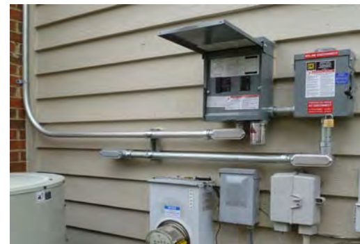
Shown here are various components of the PV solar system that monitor usage and production.
