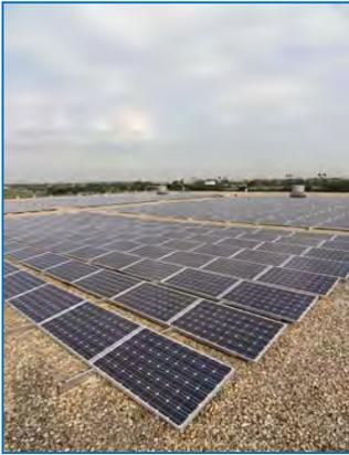
On the roof of United Displaycraft in Des Plaines is a 650-panel solar photovoltaic array that, with a grant from the state and federal tax incentives, will deliver over 25 years of electricity at less than seven cents per kilowatt hour.
