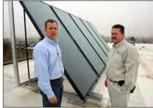
Jim Marison, left, overseer of solar systems at College of Lake County and Charlie Privett, facilities manager, stand by solar panels that are used to heat water for the building.
